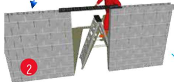
Lintel is placed in position
